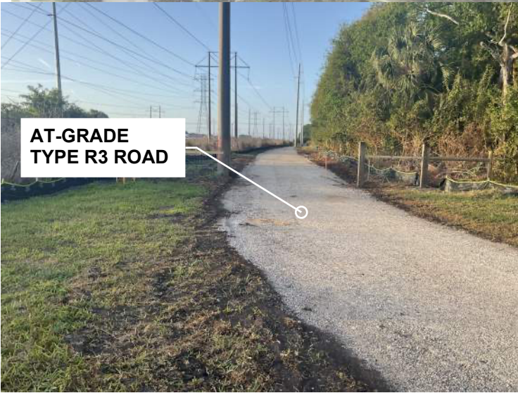
PHOTO OF COMPLETE GRAVEL ACCESS ROAD
